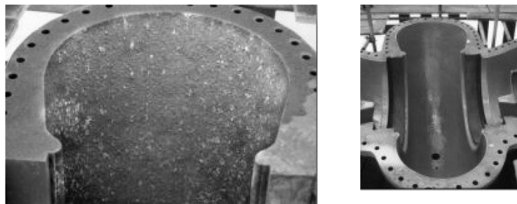
Figure 9.10 Surface of a pump casing before and after a finished coat
